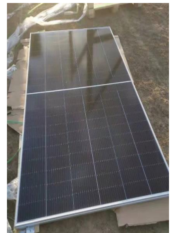
Bottom module placed on the pallets
